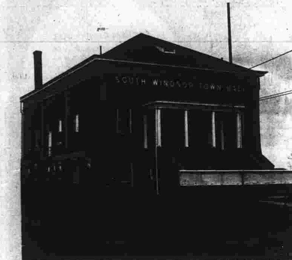
Old town hall on Main St., built in 1913, will be torn down.
