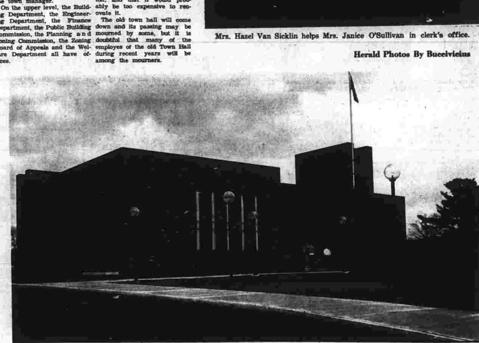
Costing over $700,000, new town hall is at Ellington Rd. and Sullivan Ave., the geographical center of South Windsor.
